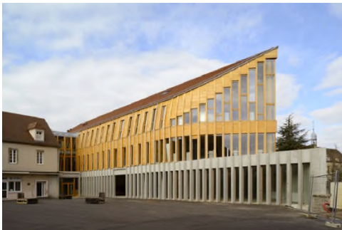
François Pompon College (1965), on the left before the 2016 extension: rough concrete base, bow-shaped lamibois structure, gable roof.
